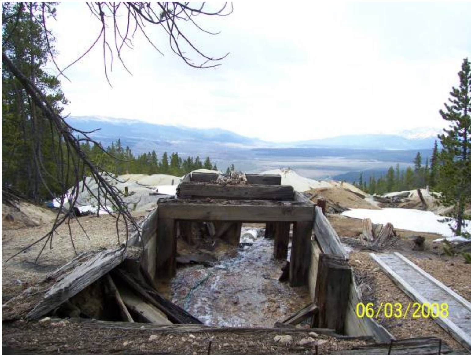
Acid mine drainage from the collapsed Tiger Tunnel runs across the large mine waste pile.
