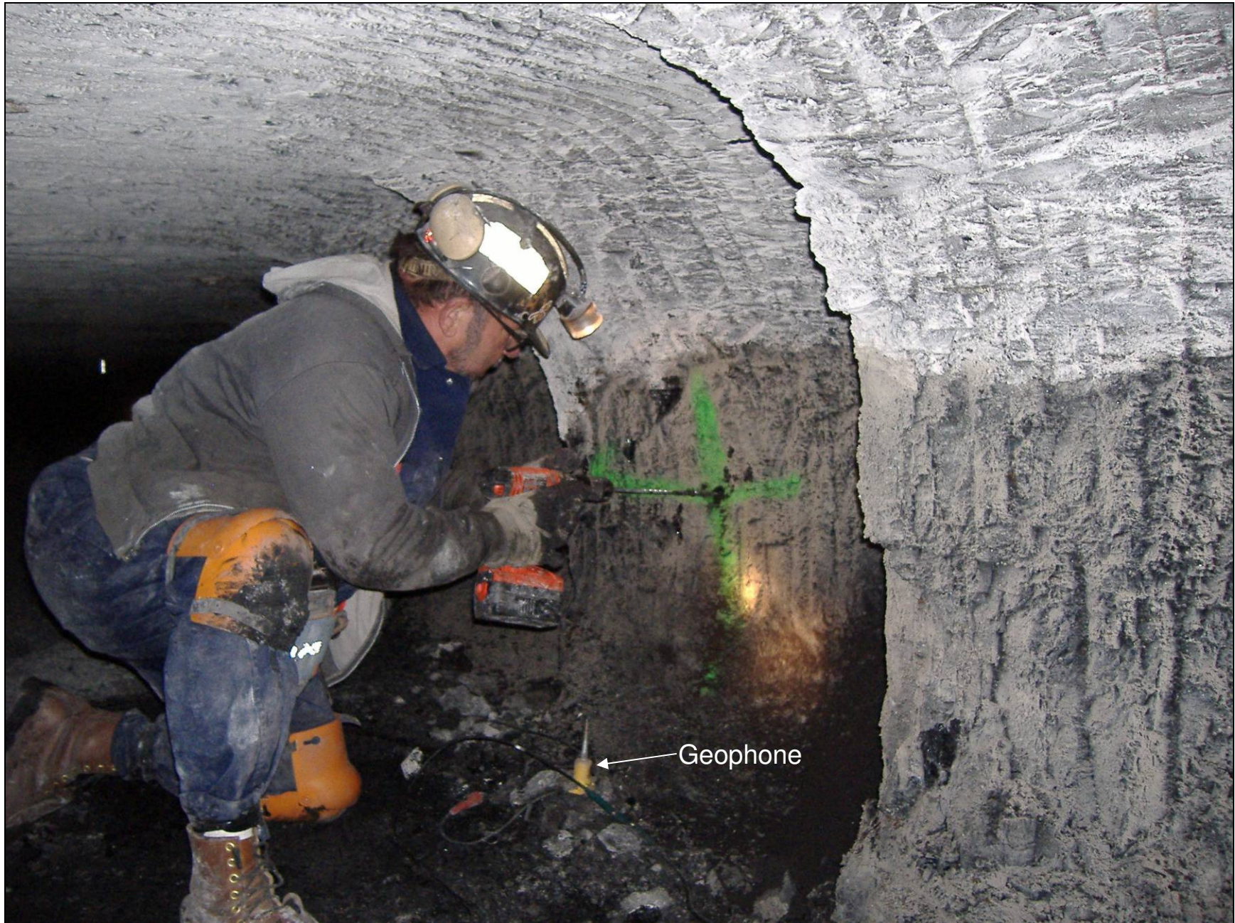
Typical geophone installation into coal rib using a cordless drill.
