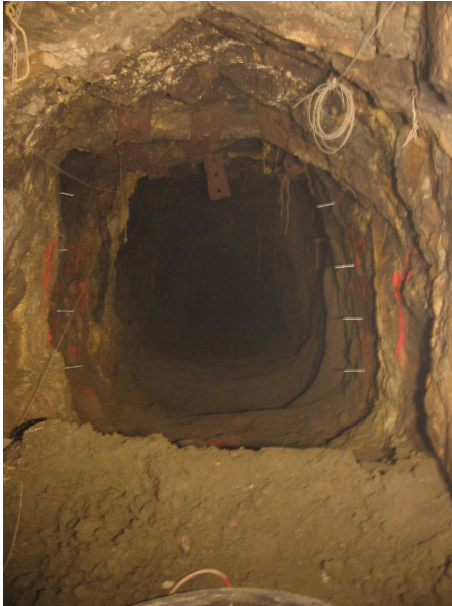
Tunnel conditions prior to bulkhead construction
