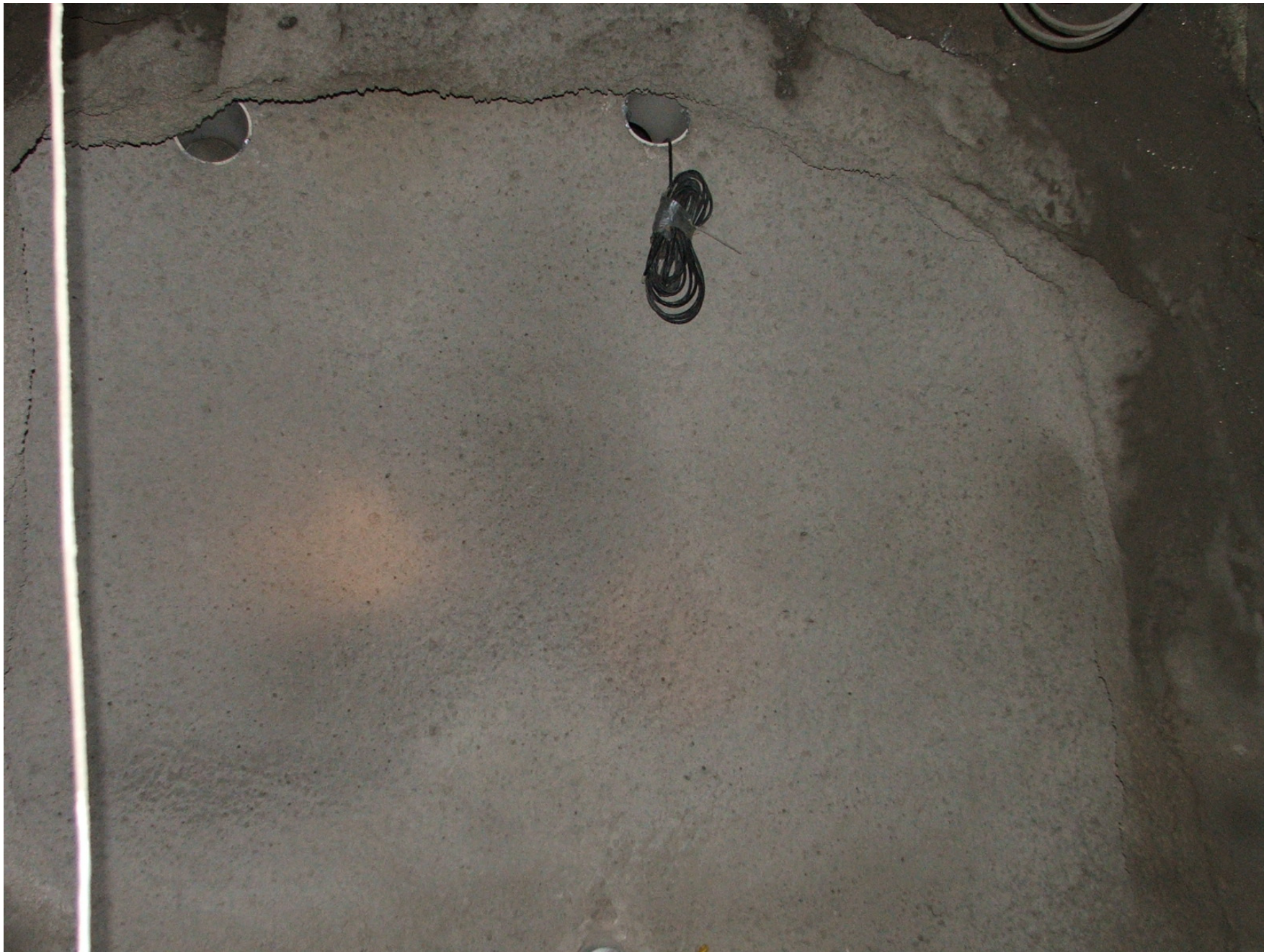
Completed reinforced concrete bulkhead
