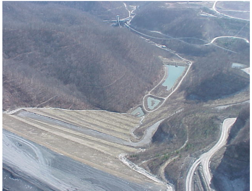
Fill and Sediment Structures
